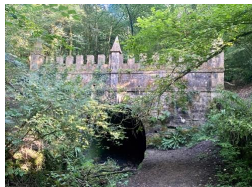
Sapperton Railway Tunnel, Daneway Portal
